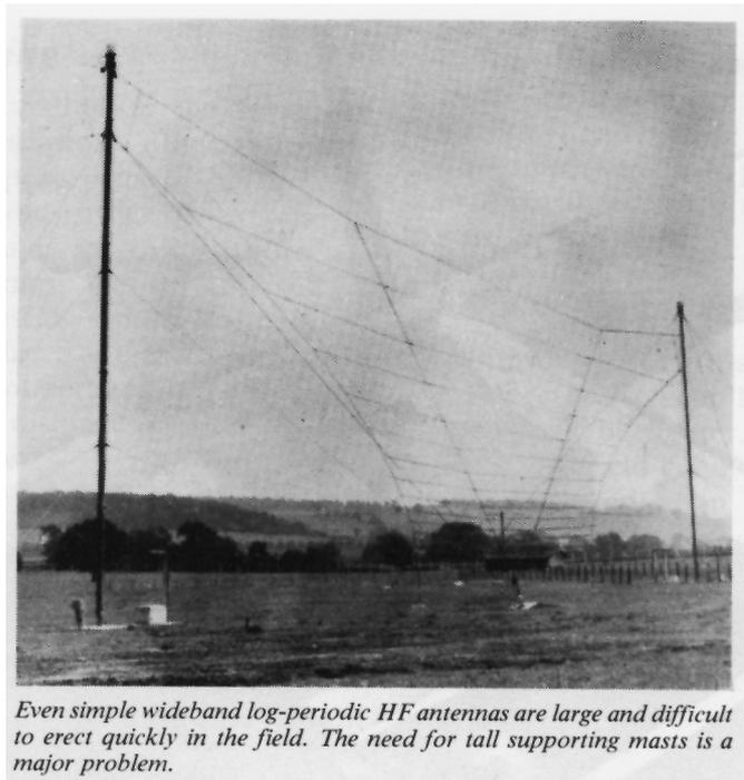
Transportable antennas usually take the form of dipoles or inverted 'L' antennas for short ranges and sloping-Vee antennas for longer paths. The major problem with high gain antennas for field use is
